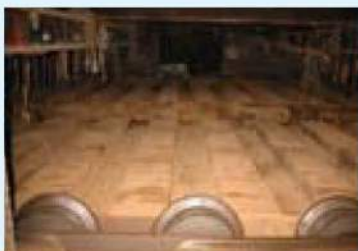
Conveyor for Bulk Waste/Recycling Facility
